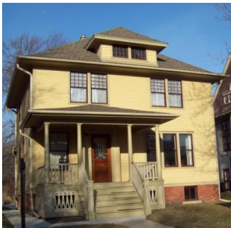
Wyandotte Museum Offices (Burns Home) 2624 Biddle Avenue Houses: Wyandotte Museum Offices & Archives, Special Event Offices, Historical Society Offices Extent of Use: Moderate
