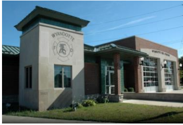
Fire Station #2 1093 Ford Avenue Houses: Fire Station Extent of Use: Heavy
