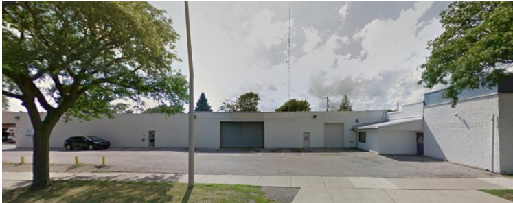
Recreation Maintenance Garage 1100 Biddle Avenue Houses: Storage for senior vehicles & equipment, parks equipment & museums archive and storage Extent of Use: High
